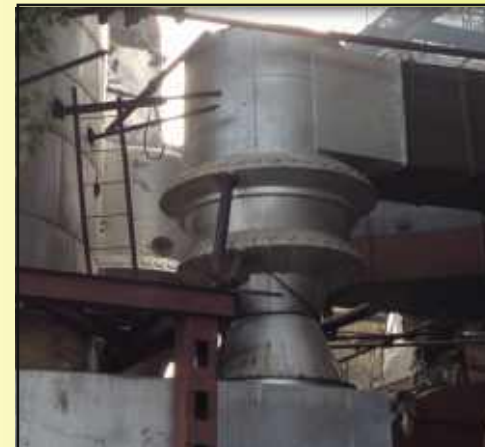
Cyclo Venturi Scrubber at one of the Sugar mills
