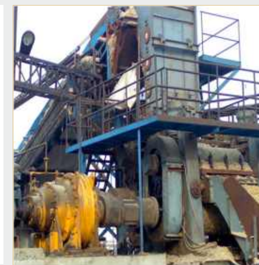
Two Roller Enmill Extraction Mill In Operation
