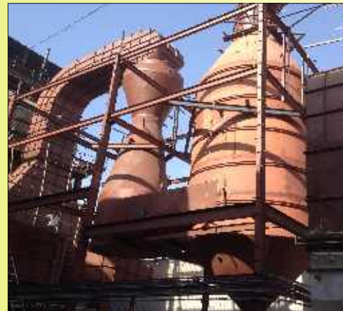
Venturi Scrubber under installation
